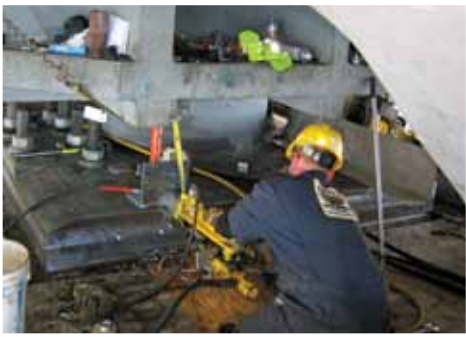
Drill Shear Key Holes
