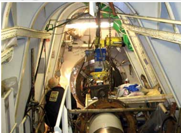
Machine Stern Tube Seal Flange
