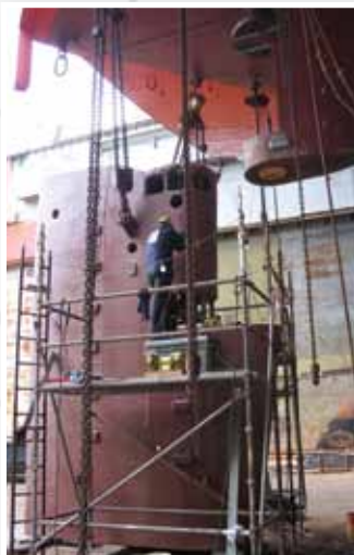
Machine Tapered Pintle Bore
