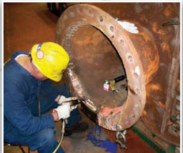
Metalstitch® Cold Cast Iron Repair
