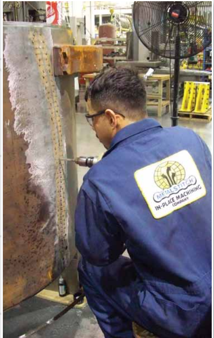
Motor Stator Metalstitch® Repair
