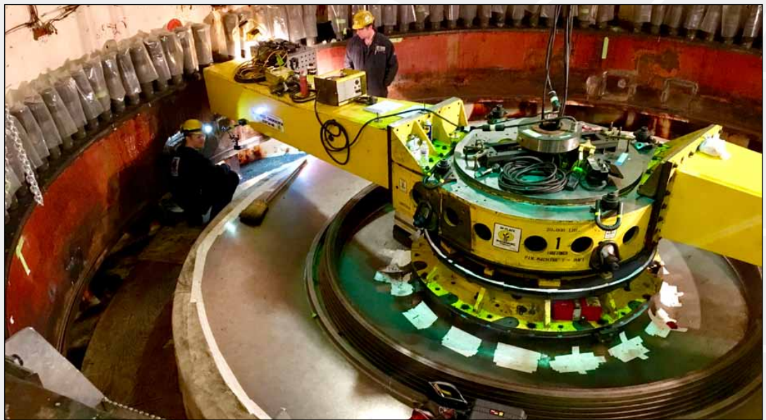
Weld and Machine Stay Ring O-Ring Groove with Pin Machine
