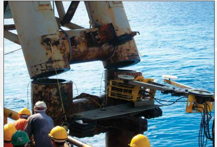
*Platform Legs Cutting with Diamond Wire Saw*
