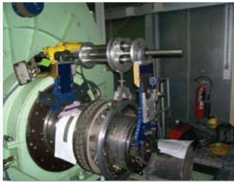
Refurbish Collector Rings
