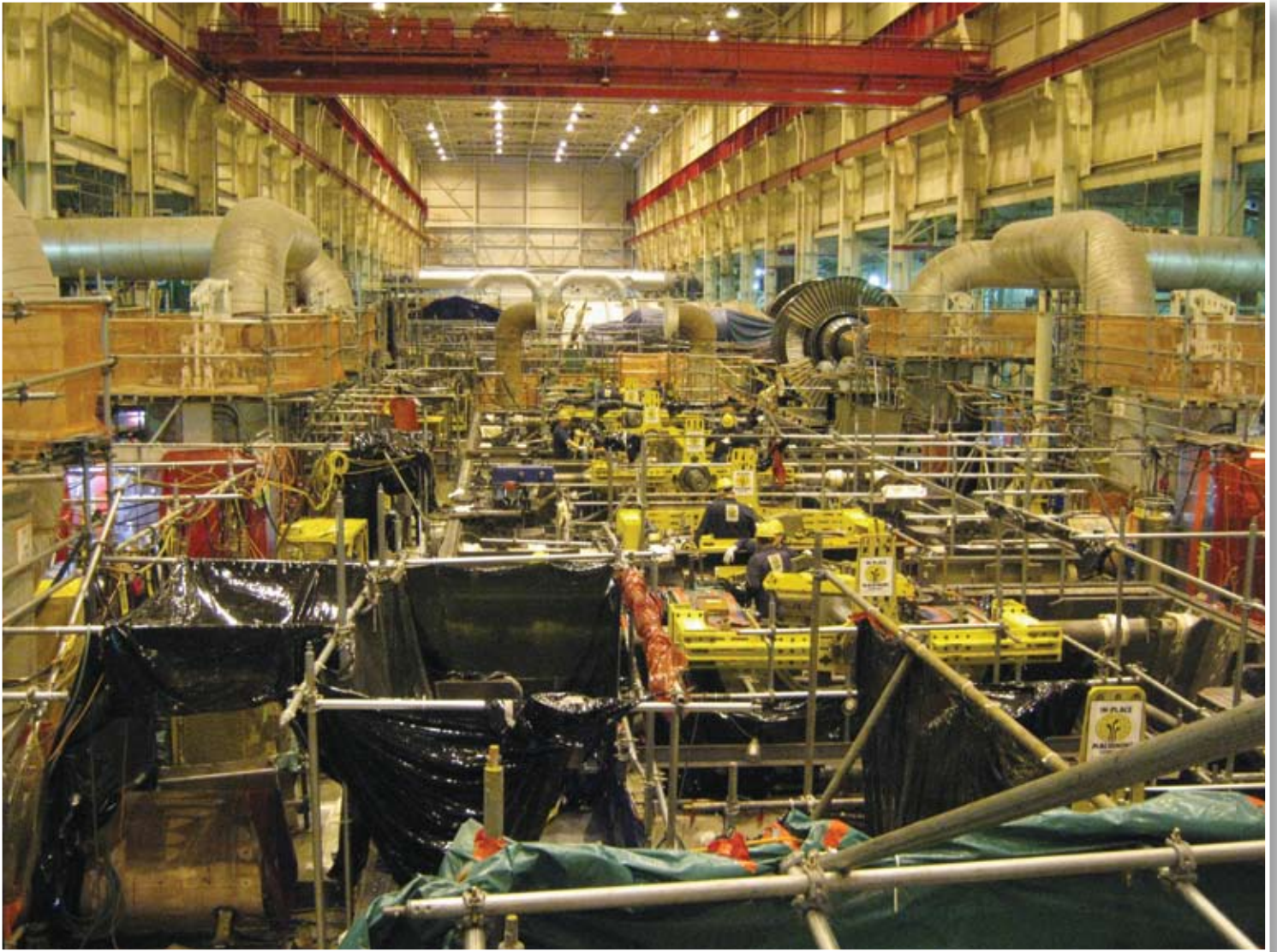
Bore 6 LP Turbine Cases Simultaneously at a Nuclear Power Plant
