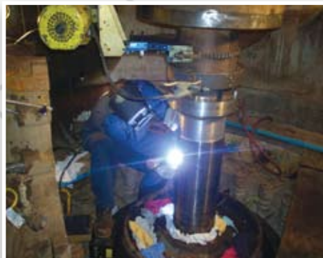
Manufacture and Install Sleeve
