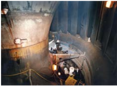
Weld Discharge Ring with Runner Installed
