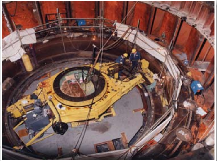
Weld Overlay and Machine Seal Ring
