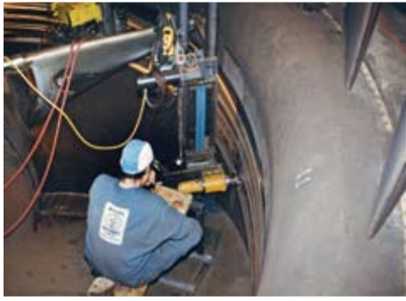
Pre-Machine Discharge Ring Before Welding
