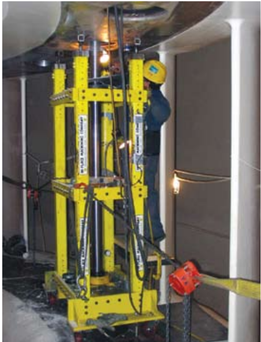
Wicket Gate Boring
