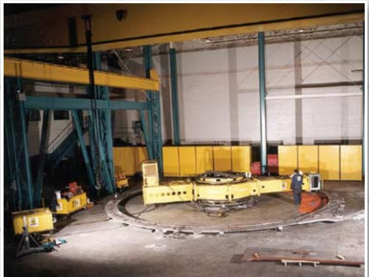
Weld and Machine 10 Meter Control Ring
