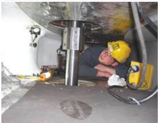
Wicket Gate Boring
