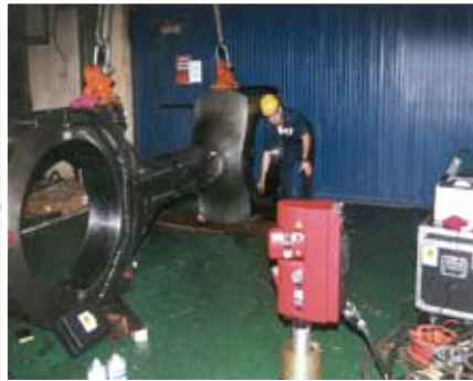
Large Engine Repair
