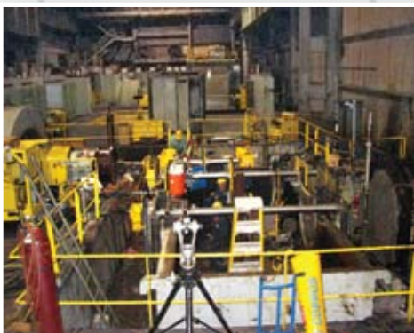
Weld and Line Bore Rough Mill Gear Box
