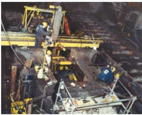
Mill Stand Refurbishment
