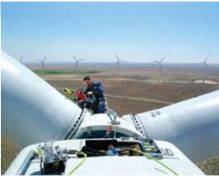
Wind Power Generation
