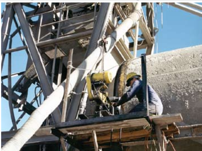
Grind Kiln Tire
