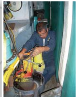
Repair and Reinforce Damaged Yaw Drive Flange
