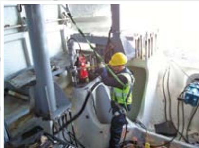
Remove Broken Studs and Refurbish Threaded Holes Up-Tower
