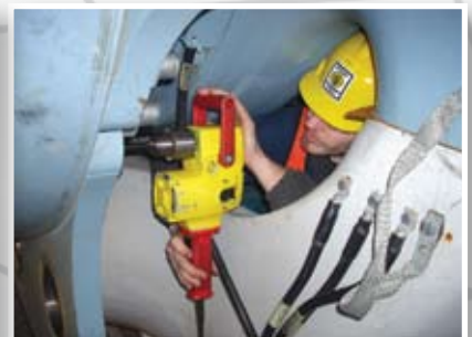
Remove Broken Studs and Refurbish Threaded Holes Up-Tower
