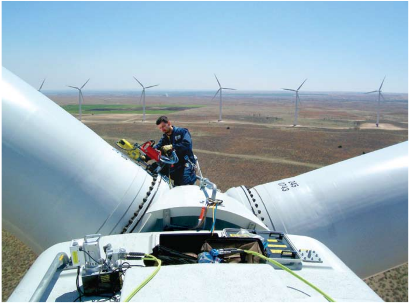
Remove Damaged Blade Studs and Refurbish Threaded Holes
