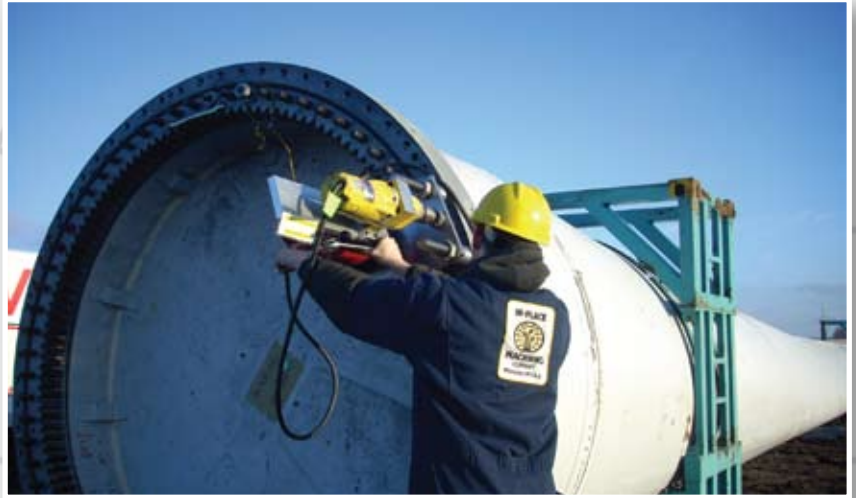
Repair Damaged Holes
