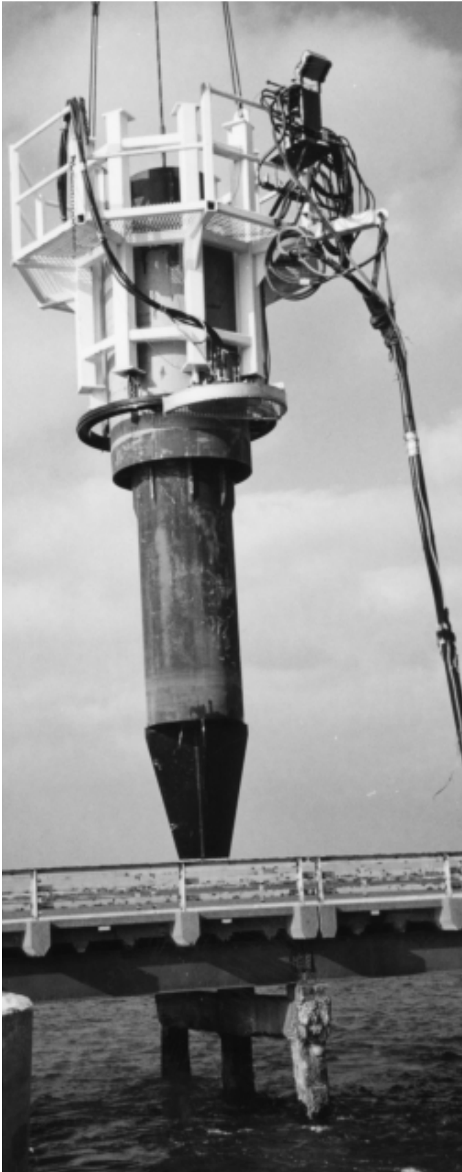
Left: The crane lines up support work platform and saw.
