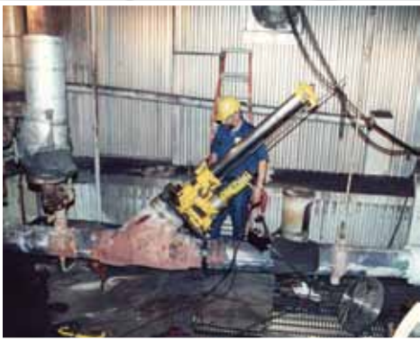
Valve Seat Machining
