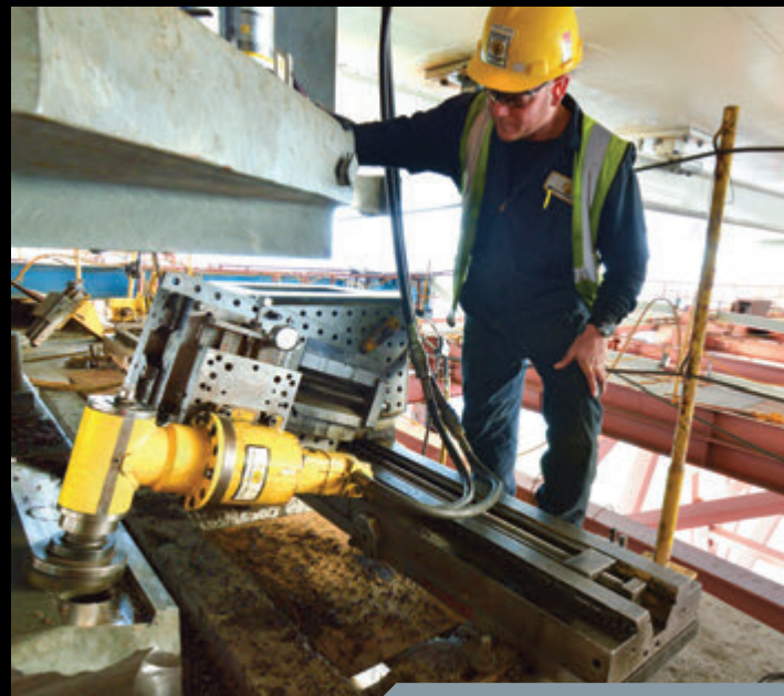
MILLING BRIDGE SHEAR KEY BASEPLATES
