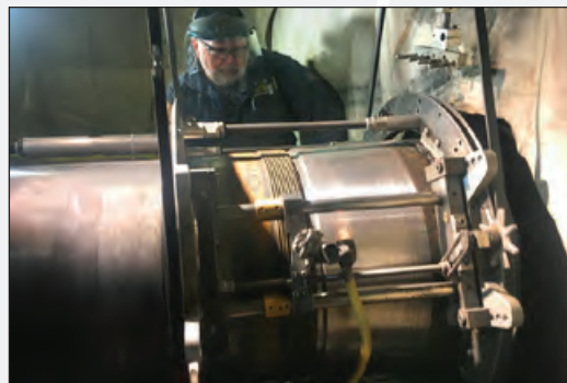
Yankee Dryer Bearing Tapered Journal Refurbishment
