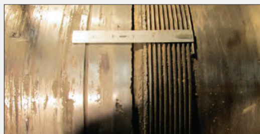
Before Repair: Deep Scoring of the Tapered Bearing Journal
