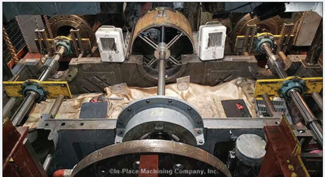
Marine Gearbox Repair Performed in the Ship
