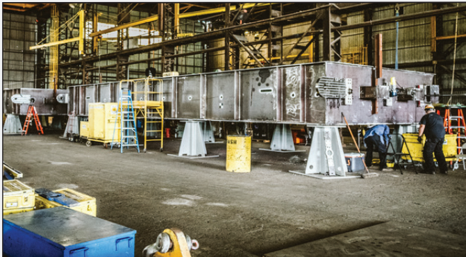
New Fabrication - McNary Dam Closure Leaves (Photo Credit TMF)
