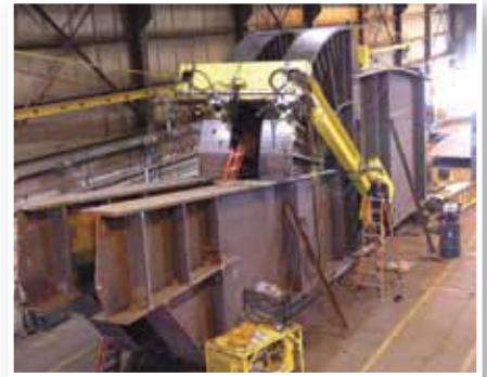
Bridge & Infrastructure Repair
