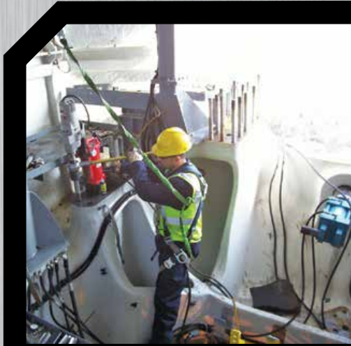
STUD REMOVAL & REFURBISH THREADED HOLES UP-TOWER
