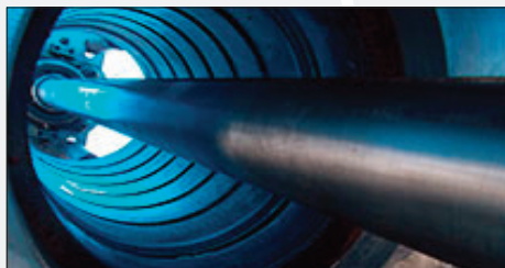
On-Site Machining with Boring Bar
