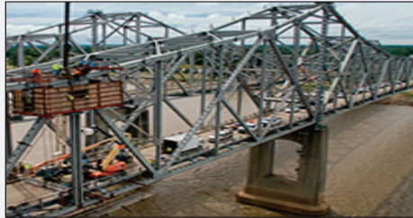
US 84 Mississippi River Bridge Repair (Photo: HNTB)
