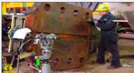
Accomplishing The Most Difficult On-Site Alignment
