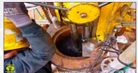
Cement Mill Grinding Table Field Machining
