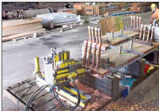
On-Site Machining Copper Staves for Blast Furnace
