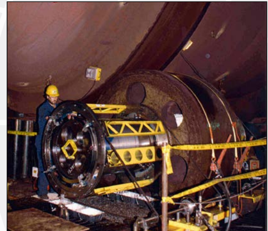
Iron Mine Pelletizing Kiln Journal Refurbishment
