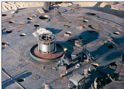
Machine Center Pin on Dragline
