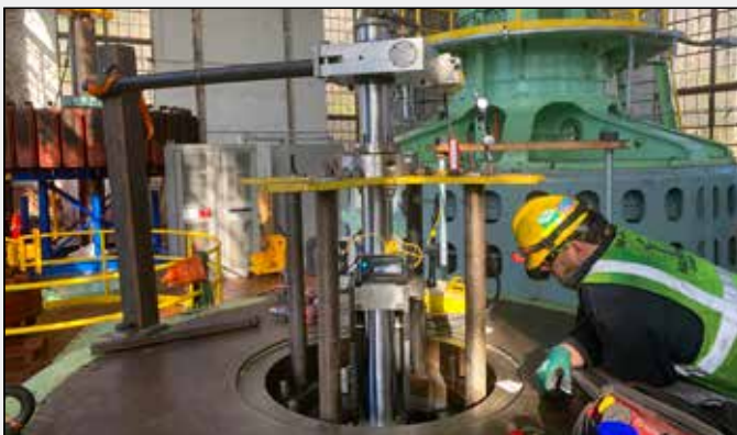
On-Site Field Machining at a Hydro Power Plant
