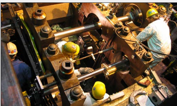
On-Site Gearbox Refurbishment
