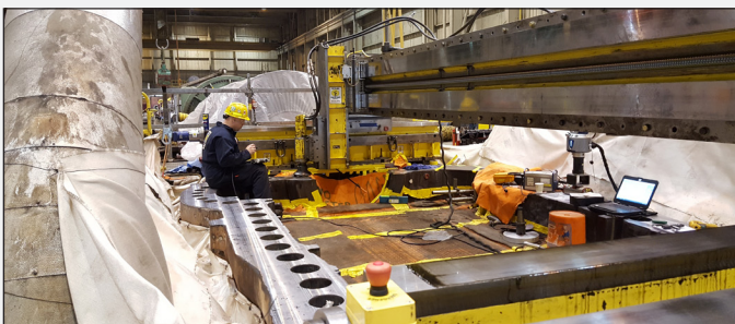
Horizontal Joint Milling On-Site
